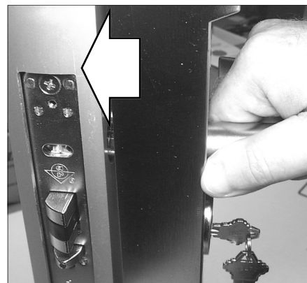
Fig. 6: Install lock onto the door
