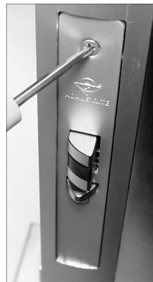
Fig. 5e: Install the latch face plate
